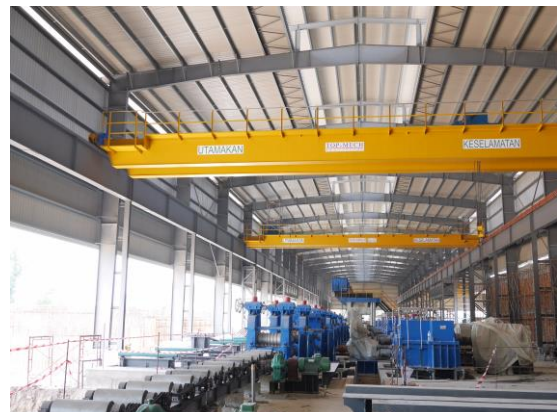
Masteel's new rolling mill in Bukit Raja, targeted to come on-stream in mid-2015
